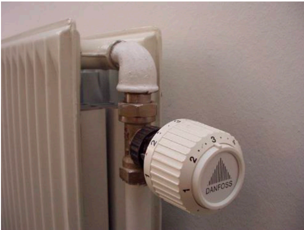
Figur 19. Radiatortermostatventil
