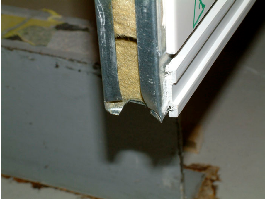
Figure 4. Corner of wall element after dynamic impact with steel ball (10 Nm).
